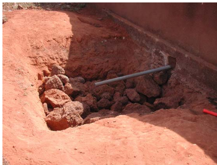
Figure 16: Open Soak Pit with Installed PVC Pipe (Ouayerma, Mali)
