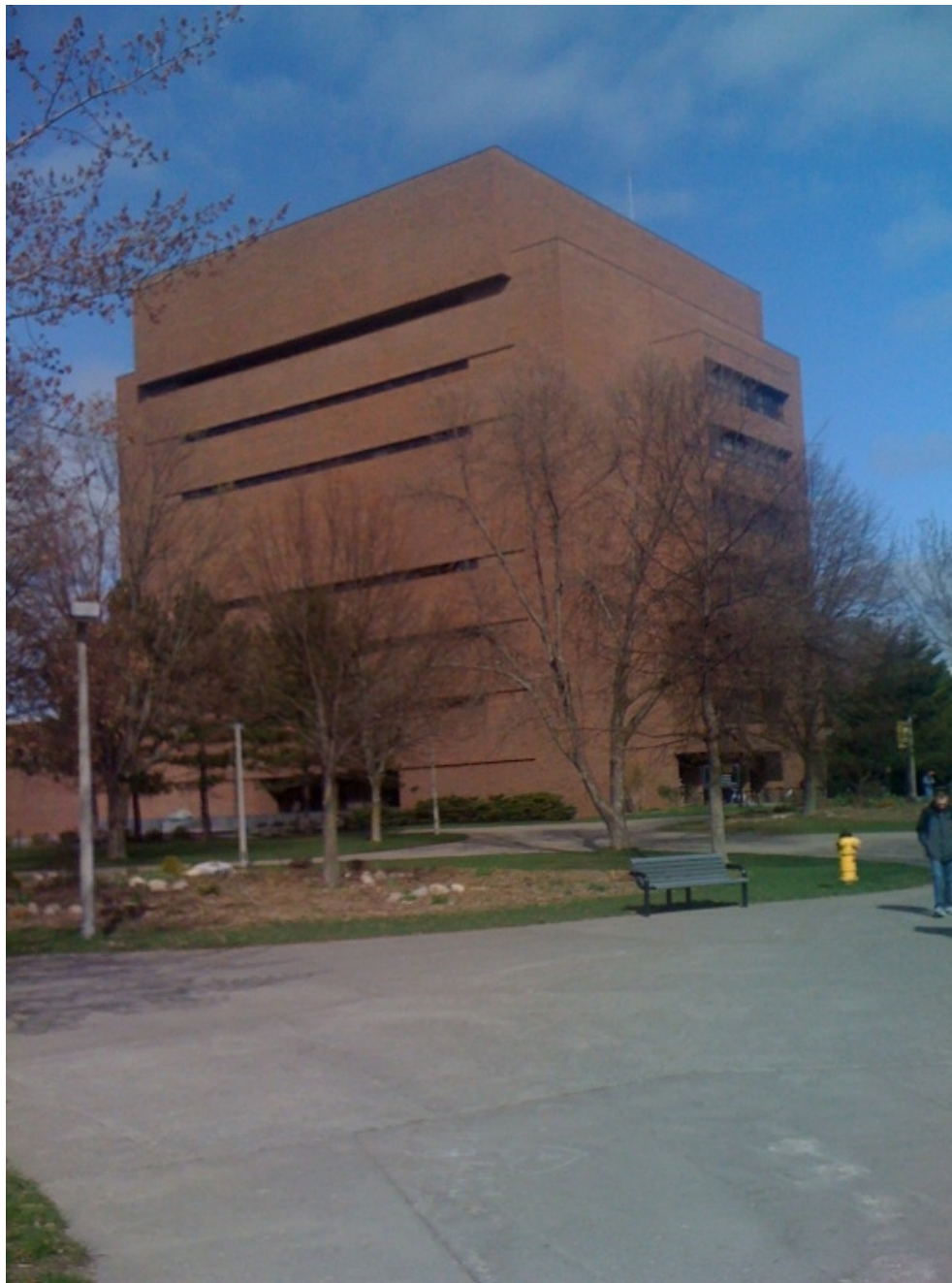
Electrical Energy Resource Center - A. E. Seaman Mineral Museum
