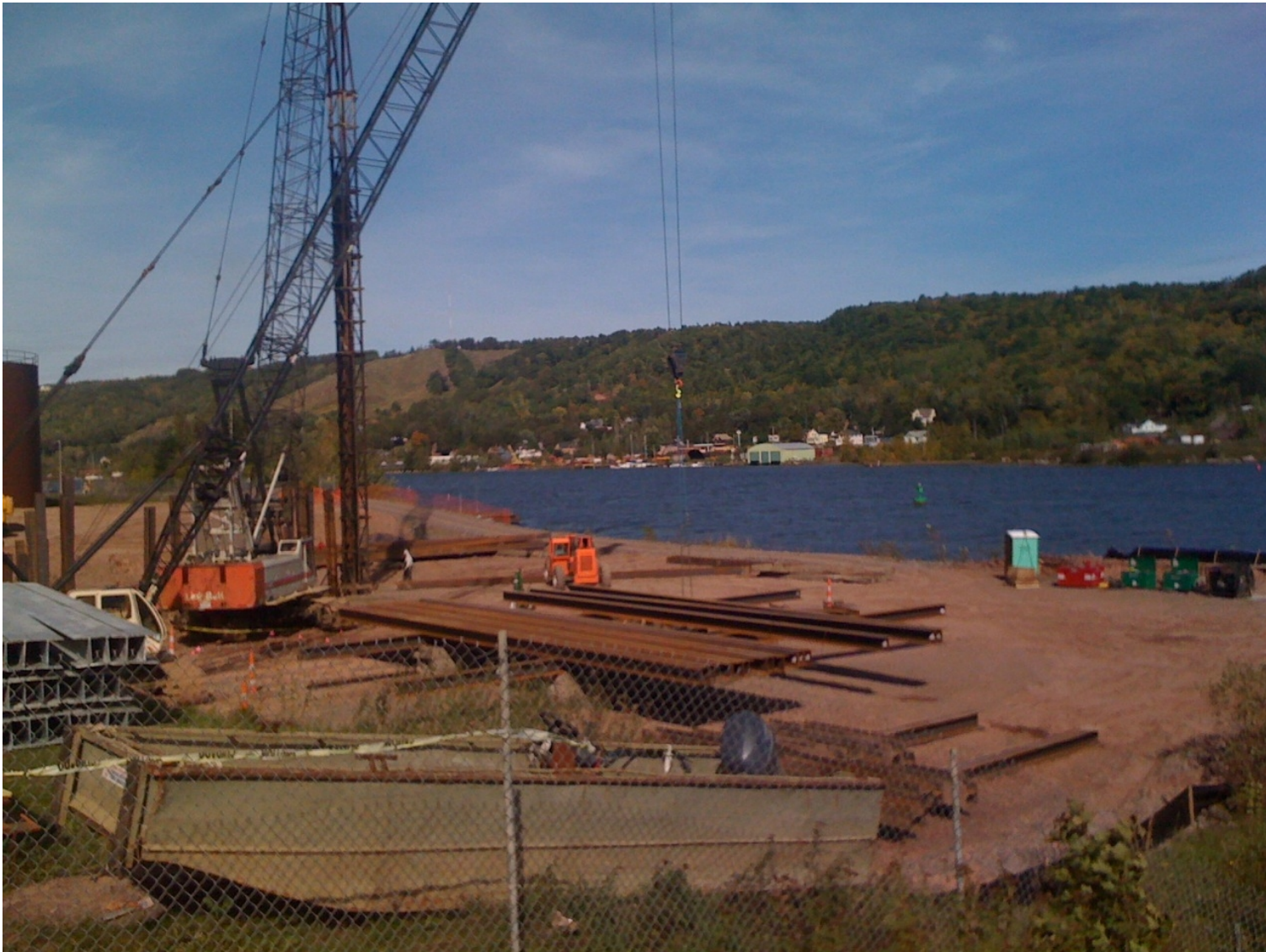
Building Site – Great Lakes Research Center
