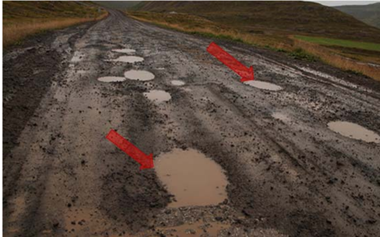
Figure 2-1: Potholes on an unpaved road.
