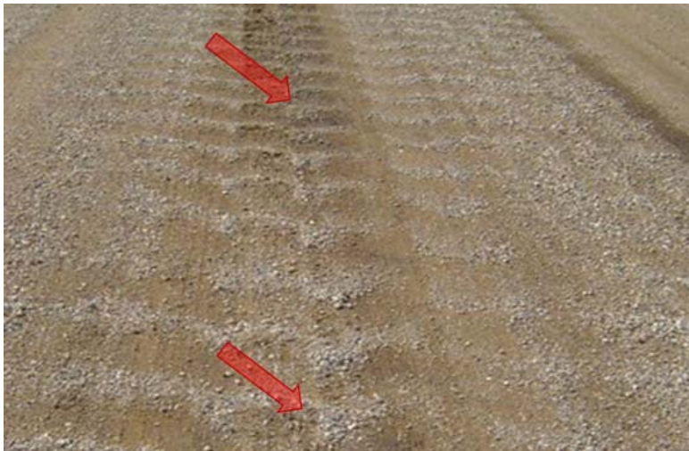
Figure 2-2: Loose aggregate on an unpaved road creates a distinctive pattern.
