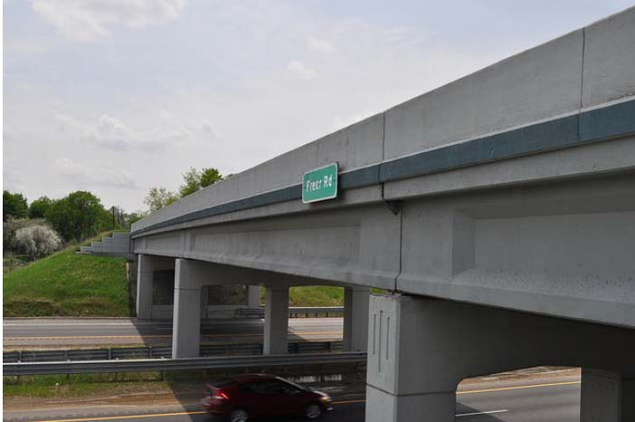
Figure 2: MDOT structure n° 10940, Freer Rd over 1-94
