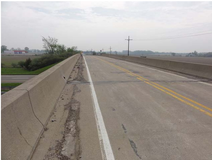
Figure 3: MDOT structure n° 10892, Willow Rd over US-23
