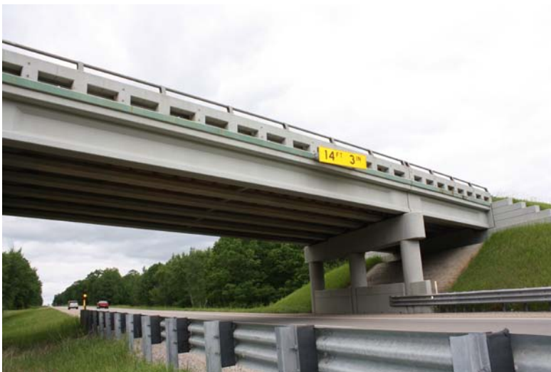
Figure 4: MDOT structure n° 1713, Mannsiding Rd over US-127 NB
