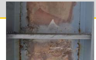
Spalls located under the bridge deck.
