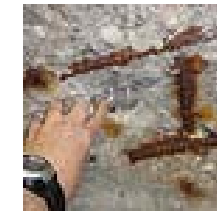
Deck Section Loss
