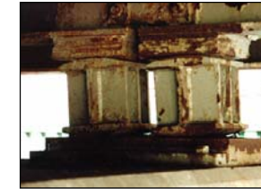
Deteriorated Bearing
