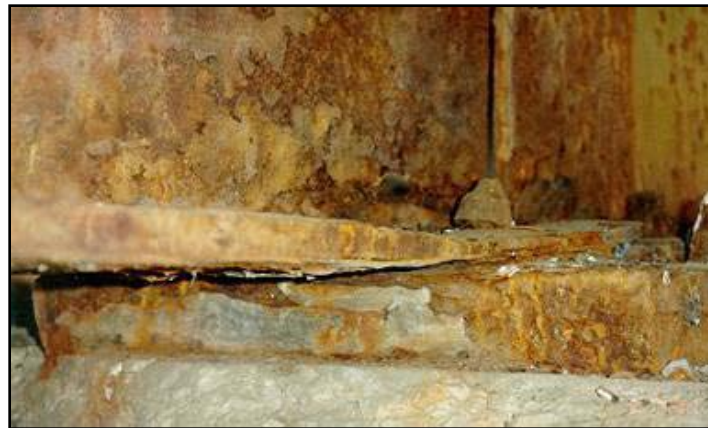
Corrosion and Section
