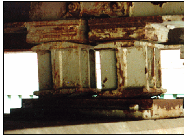
Deteriorated Bearing
