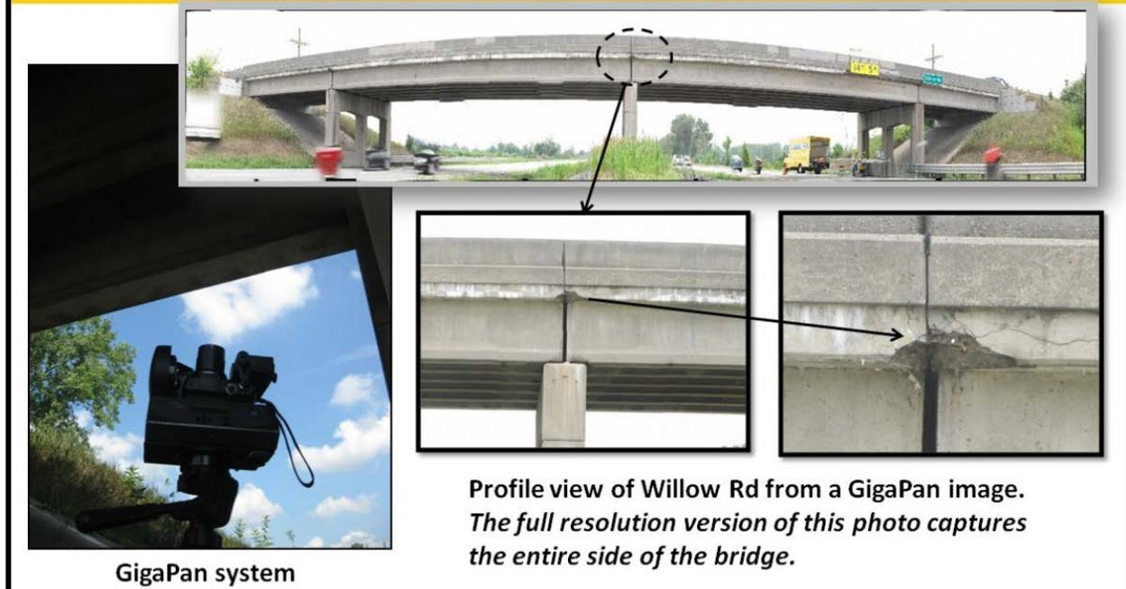
Figure 6-3: An example of the GigaPan image of a bridge fascia at the Willow Road bridge. The image is available online at [gigapan.com/gigapans/96672](http://gigapan.com/gigapans/96672) where areas can be zoomed in on easily by end users. The EPIC robotic photo-taking hardware can be seen on the lower left.
