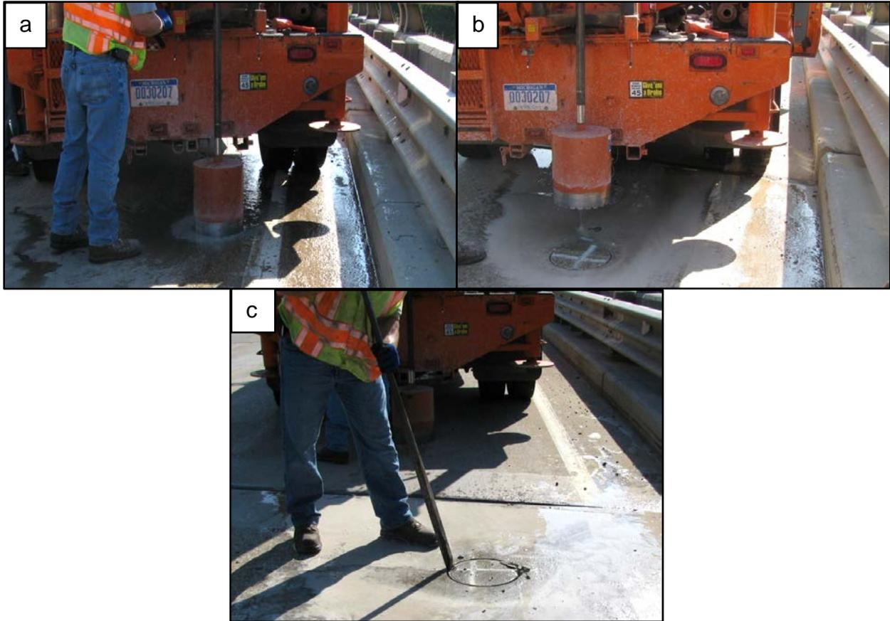
Figure 8-21: Drilling a core on the bridge deck (a), pulling out the drill (b), and pulling out the core with a pry bar (c).
