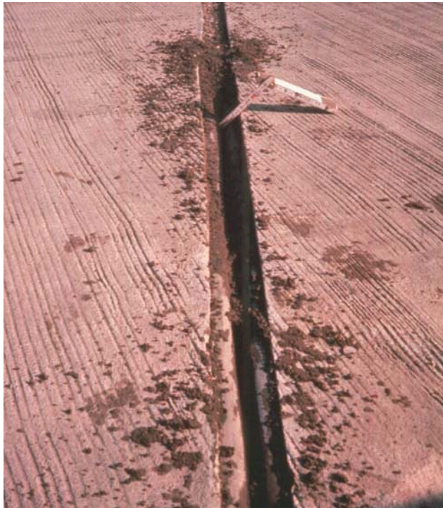
Figure 8: Material in expansion joint (FHWA 2006)
