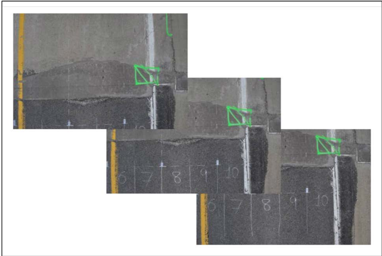
Figure 4: Photos of Willow Road bridge taken with the 3DOBS showing a 60% picture overlap for photogrammetric image creation.
