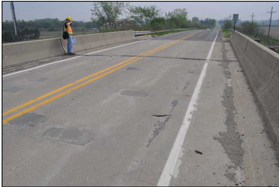
Figure 6: An example photo of the bridge deck of the Willow Road bridge taken on May 13, 2011 (note the variety of visible deck surface defects).
