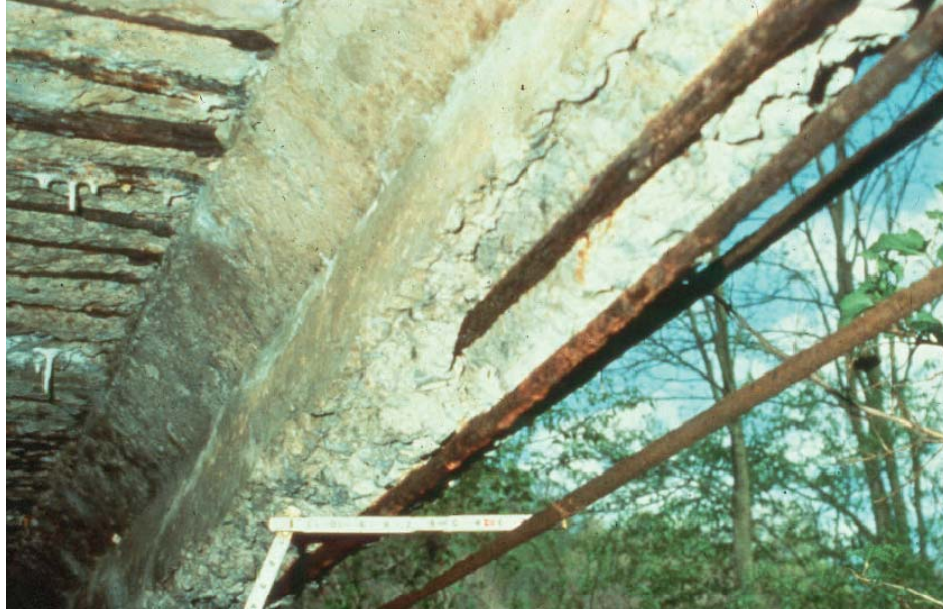
Figure 14: Corroded reinforcing bars
