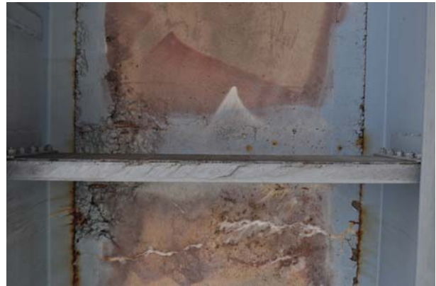
Figures 5a & 6a: Researcher taking photos of the underside of 6 Mile Bridge at US-23 near Brighton, MI. The distance from the camera to the spalls was approximately 2.5 meters (8 feet). Photo taken of spall on deck bottom surface from the field test shown above at 6 Mile/US-23 Bridge.
