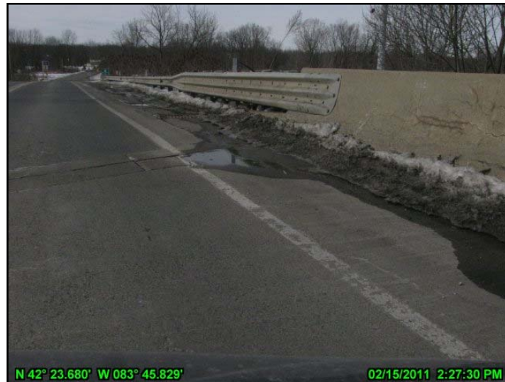
Figure 2b: A GPS-tagged photo created when driving over the 6-Mile over US-23 bridge using the BridgeViewer Remote Camera System.
