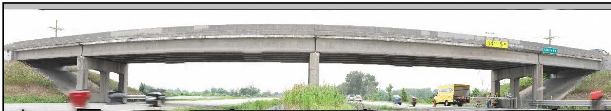
Figure 16: Profile view of Willow Road bridge looking south along US-23 from a GigaPan image. The full resolution version of this photo captures the entire side of the bridge at very high resolution in a gigapixel image.
