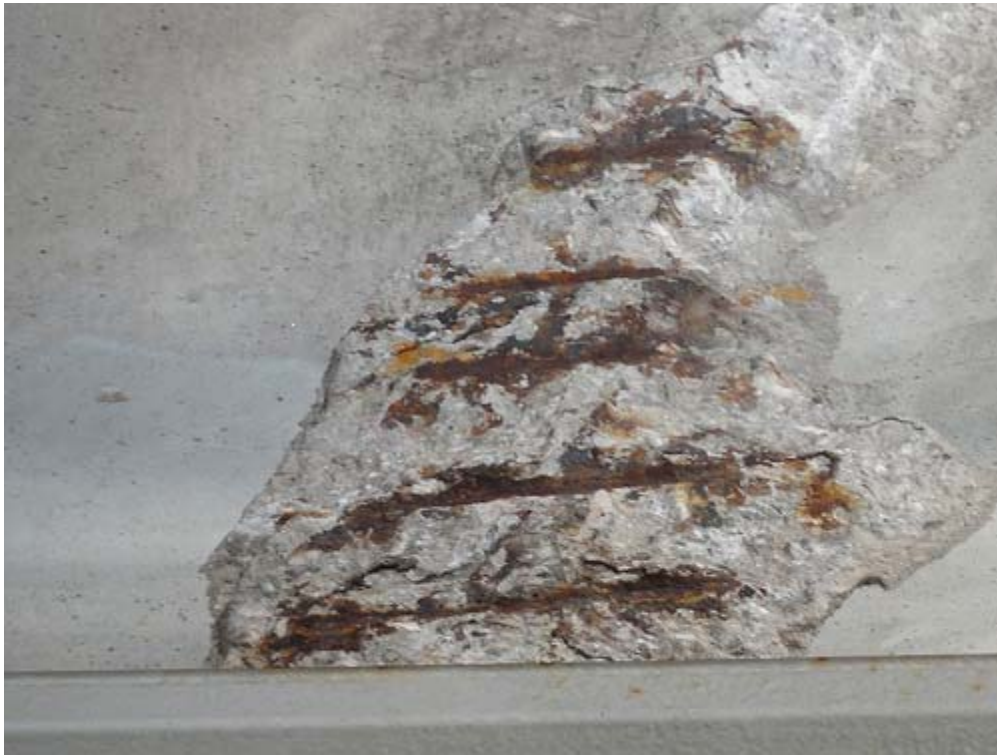
Figure 10: Corroded reinforcement in bridge deck
