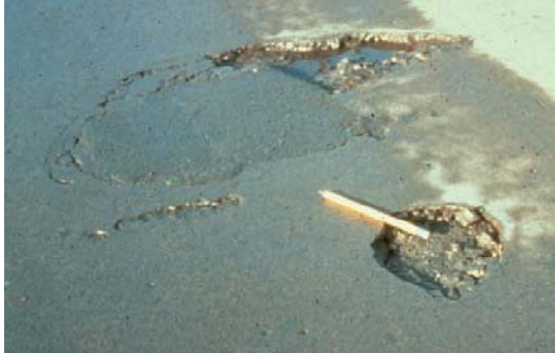
Figure 6: Concrete deck surface scaling (FHWA 2006)
