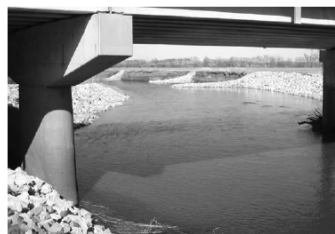
Figure 10-11. Spur dike installation along the outside bank upstream of an approach channel to a bridge.
