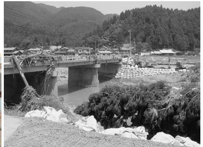
Geobags used to form and protect recently damaged abutment.
