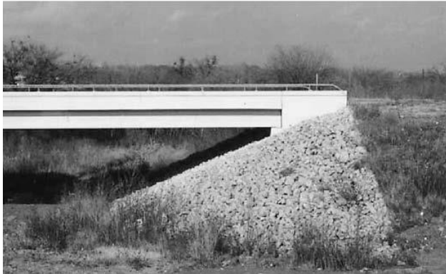
Spill-through abutment
