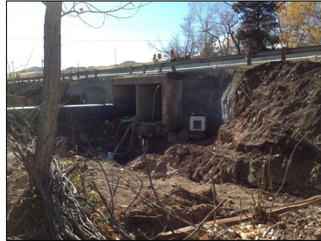
Bridge scour after overtopping event (image source: CODOT, 2017)
