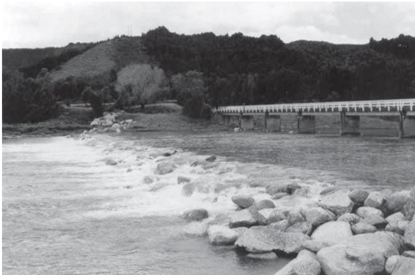
Downstream weir to arrest head-cutting
