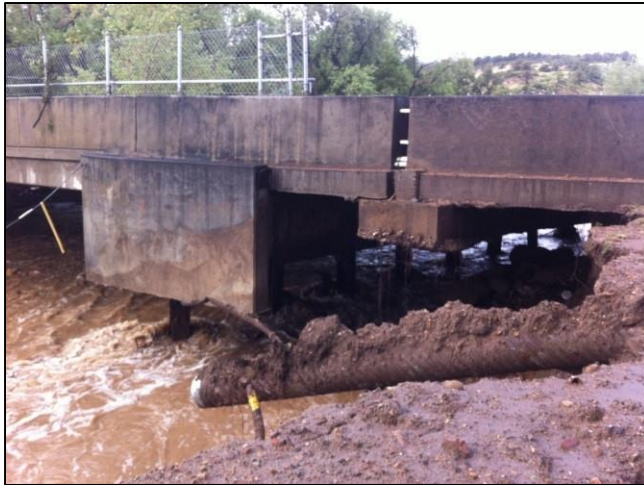
Bridge scour after overtopping event (image source: CODOT, 2017)
