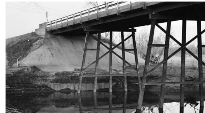
Sheet pile skirt
