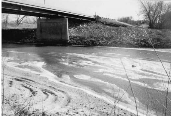
Pier very close to abutment
