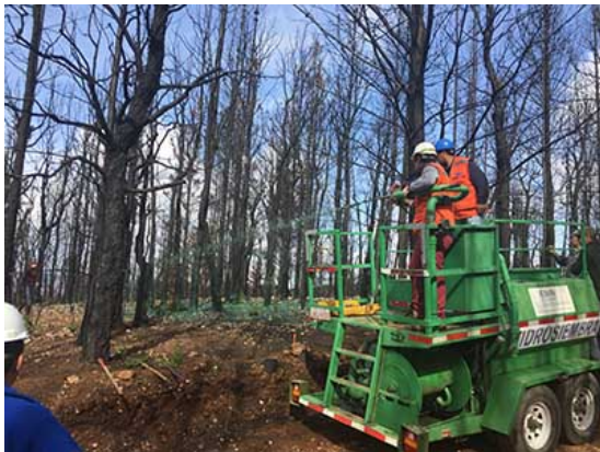
Hydro-seeding, International Erosion Control Association
