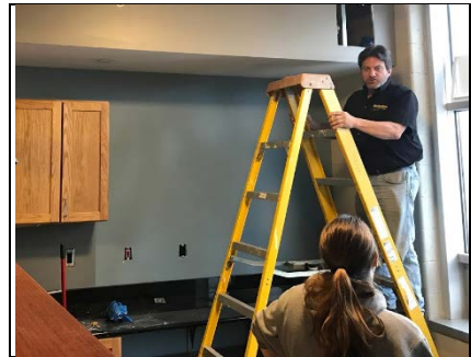
Maintenance employees making repairs on a Daniell Heights apartment.
