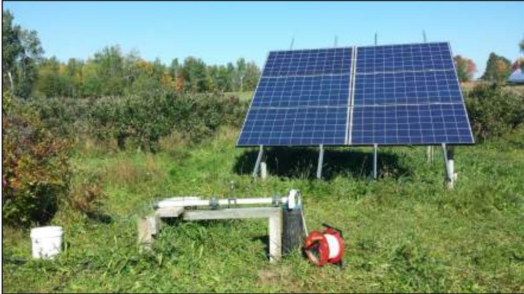
Figure 10: Solar pumping set-up at Gierke Blueberry Farm, September 2014
