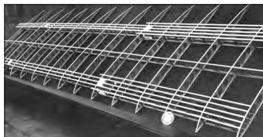
By 1919, FPL researchers were demonstrating the strength of internal web construction of an all-veneer wing.
