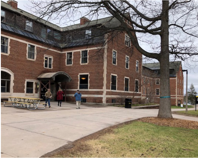
DOUGLASS HOUGHTON HALL EXTERIOR
